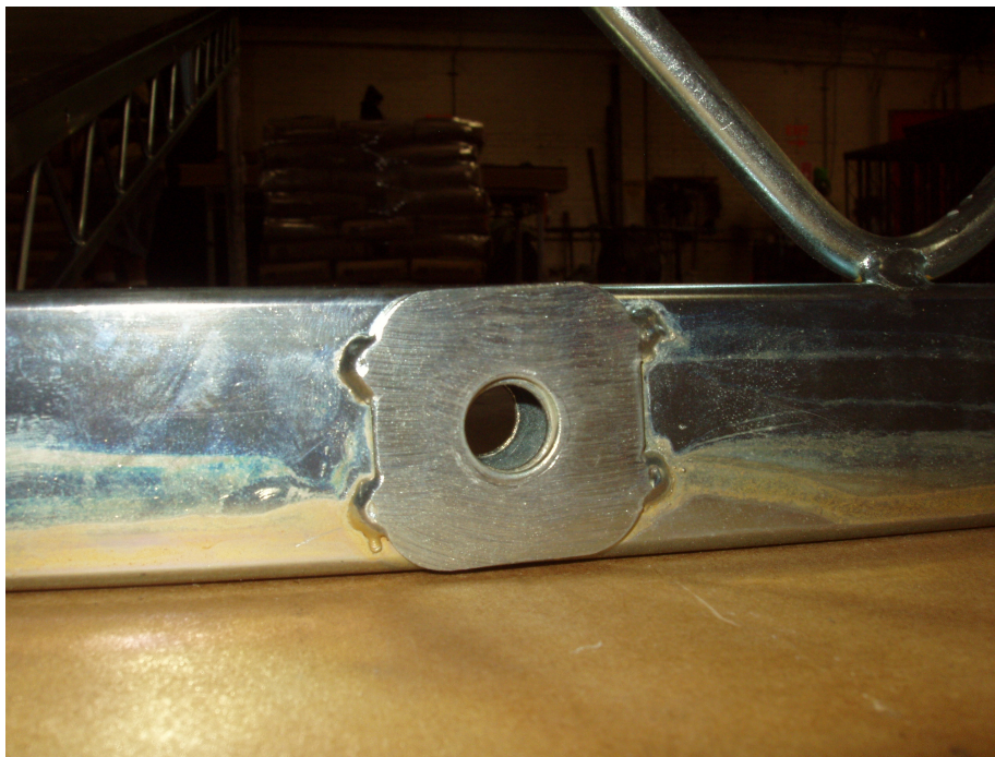
Figure 3-8 No distress of critical deck-to-deck bearing surfaces
