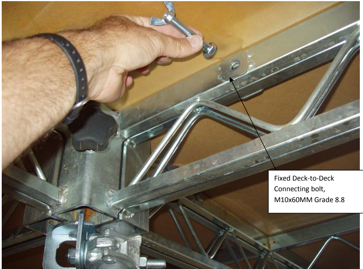
Figure 1-4 Typical STEELDECK® Deck-to-deck Connecting Bolt Joint
