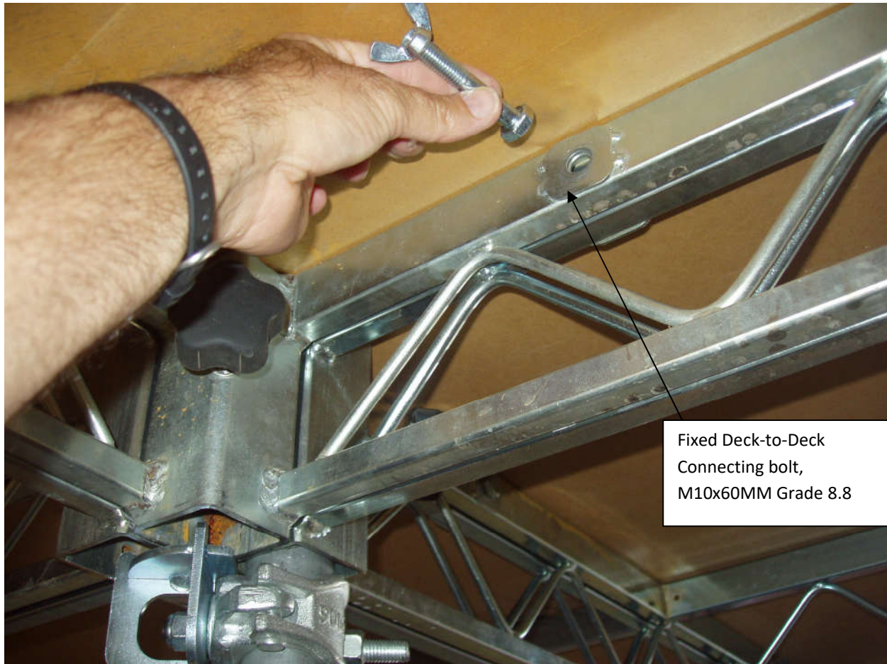
Figure 1-4 Typical STEELDECK® Deck-to-deck Connecting Bolt Joint
