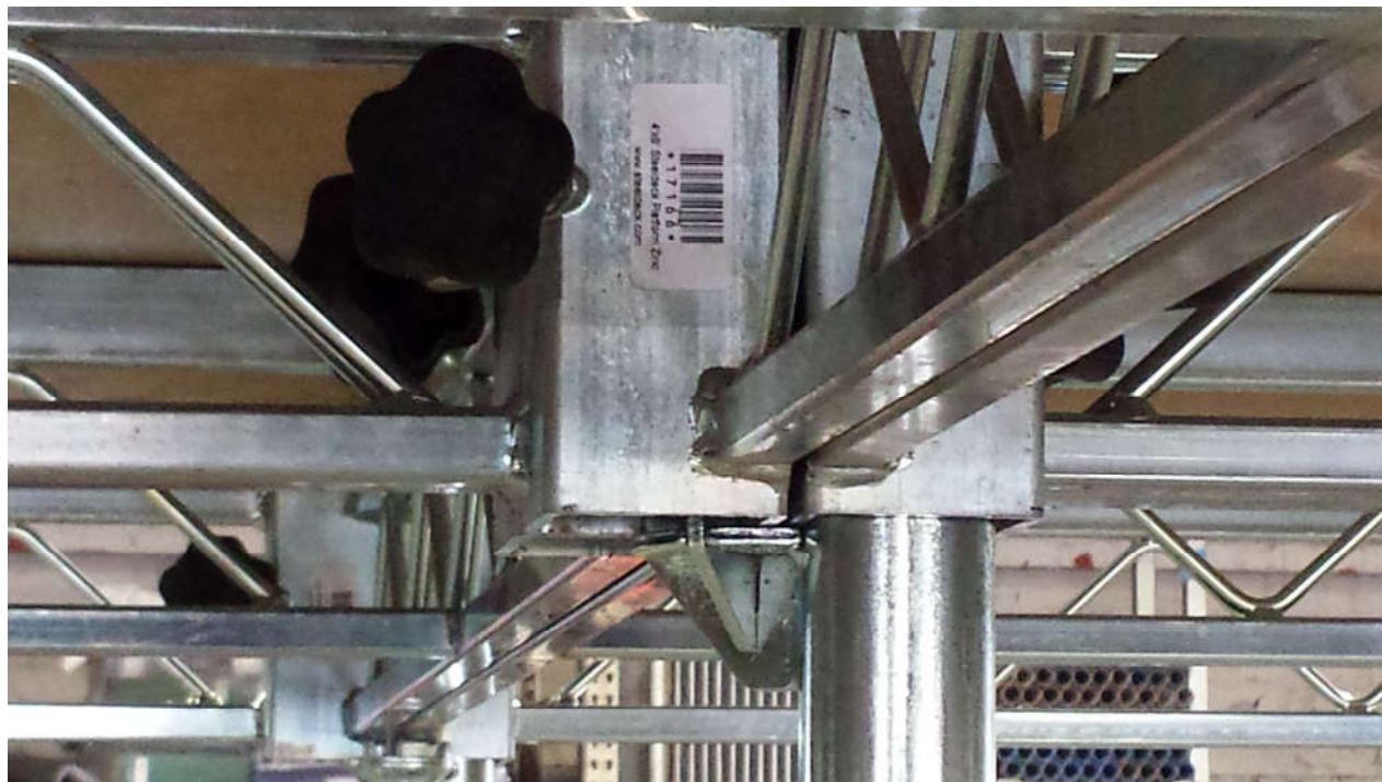
Figure 3-7 No distress of critical leg-to-deck support mount
