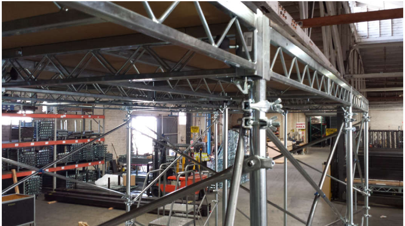
Figure 2-3 Test Platform, 10 ft high, Long View from below
