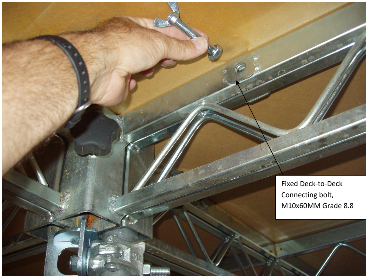
Figure 1-3 Typical STEELDECK® Deck-to-deck Connecting Bolt Joint
