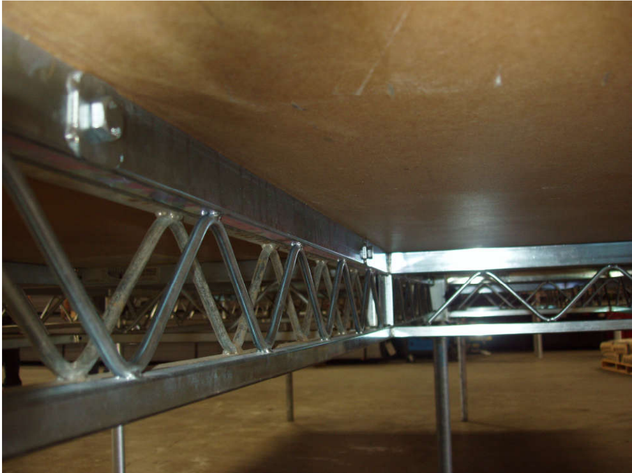
Figure 3-5 Load Step 2, 1 st Platform loaded to 271.0 lbs/ft 2 , Inboard long beams
