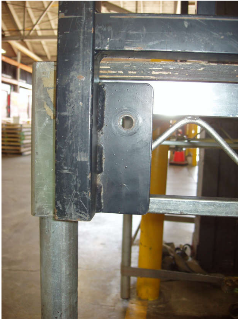
Figure 3-9 Guardrail bottom joint after tests #1-3
