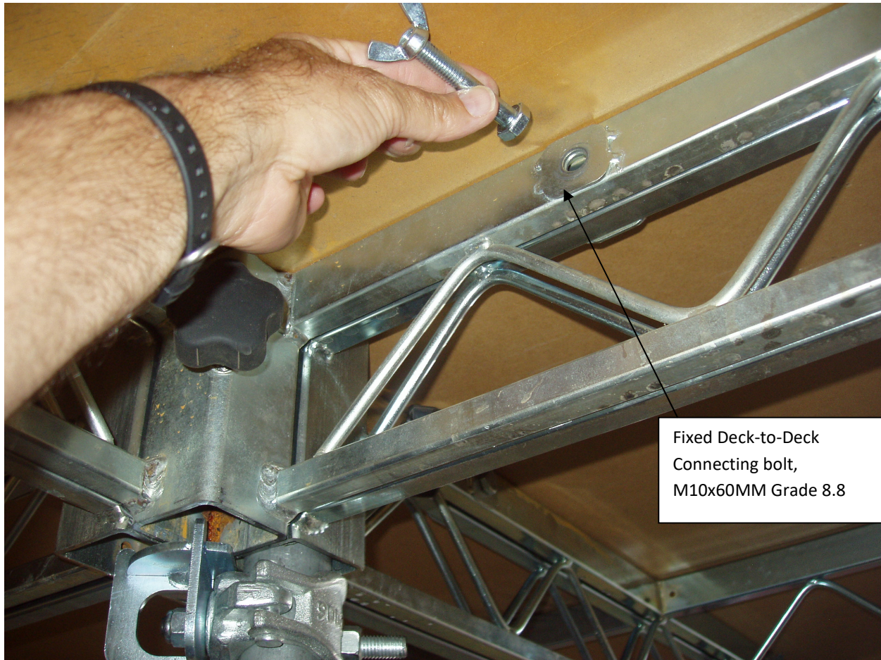
Figure 1-3 Typical STEELDECK® Deck-to-deck Connecting Bolt Joint
