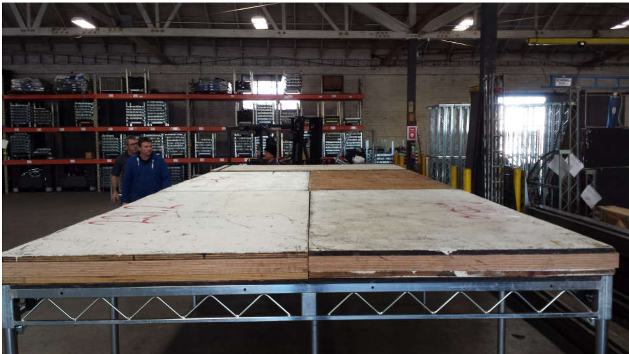
Figure 2-8 4 ft. tall 8x20 ft. Platform with wooden pallets in place, overlapping deck seams
