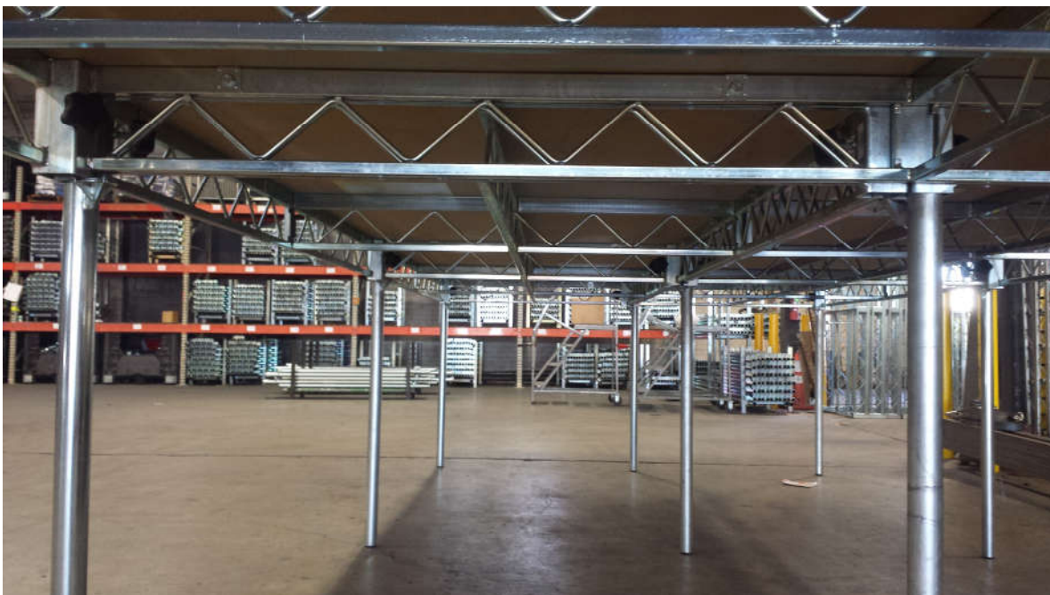
Figure 2-3 Test Platform, 4 ft high, Long View from below
