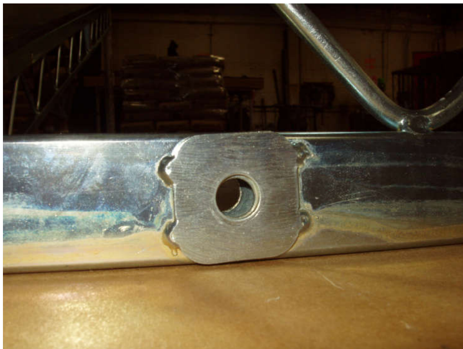
Figure 3-8 No distress of critical deck-to-deck bearing surfaces
